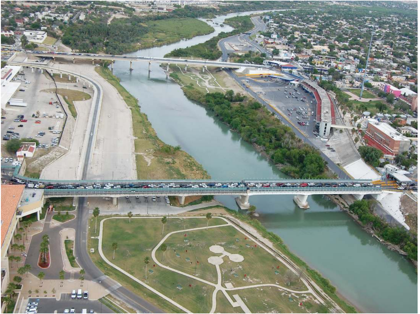
Bridge I and II in Laredo, TX
